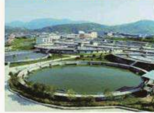
Sewage treatment plant
